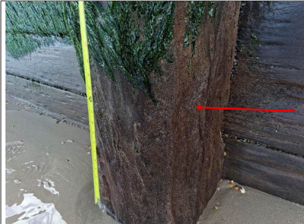
Plate 15 - Groyne C36. Gribble attack and abrasion observed on pile 5 and the plank adjacent to the landward face of the pile (indicated). This image highlights the variable performance of basralocus in the intertidal zone. The general grazing pattern over the pile, particularly the landward face results in a visual assessment rating of '3'.
