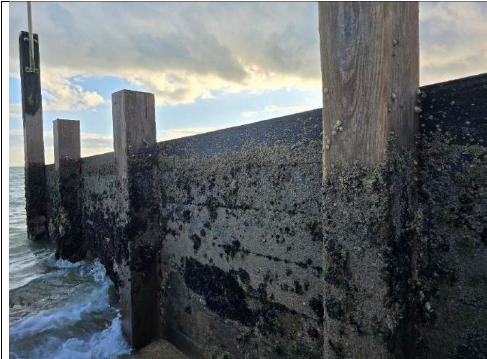
Plate 25 - Groyne 37. Seaward end of the groyne showing piles 1 to 4. Note the contrast between the paler greenheart piles and darked ekki planks.
