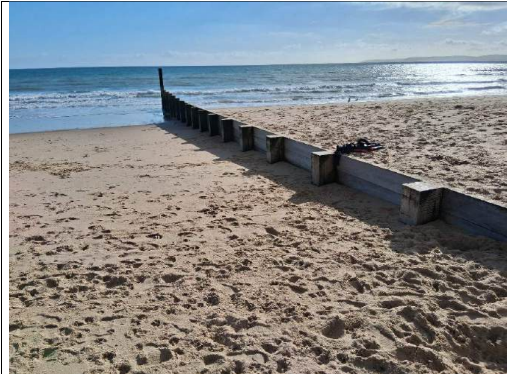
Plate 2 - Groyne C36. General appearance viewed from the downdrift side, illustrating the difference in beach levels between updrift/downdrift faces of the groyne
