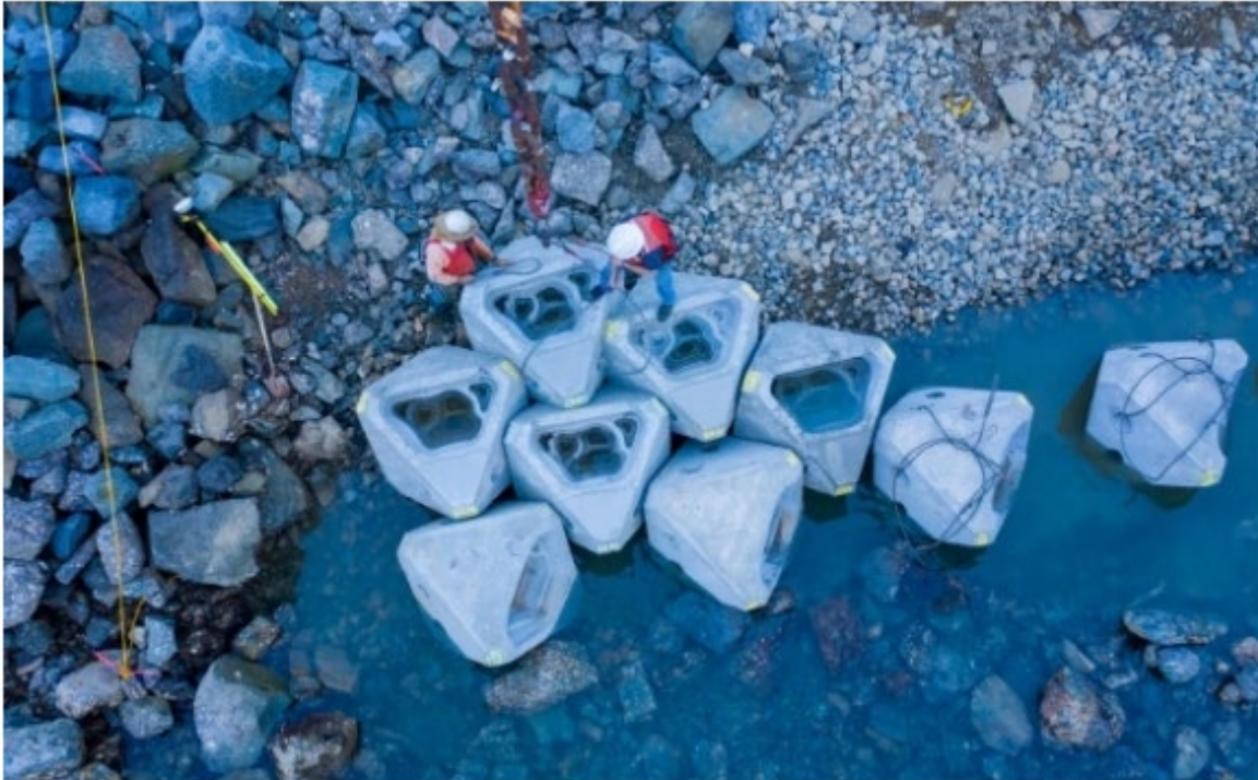
Figure 4-3 Interlocking unit constructed in San Diego (ECONcrete, 2020c).
