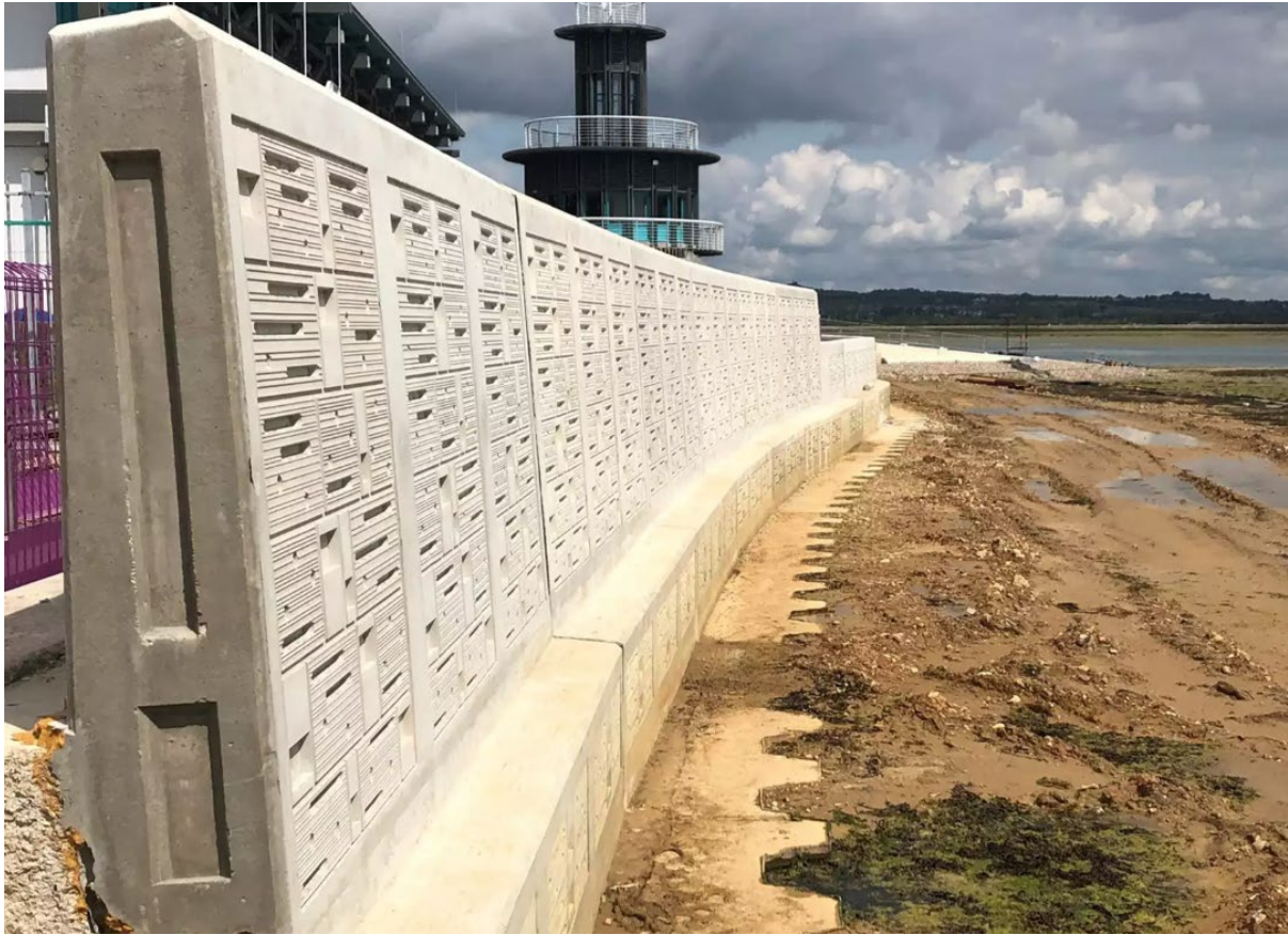
Figure 4-3 Ecoformliner Wall Curve at the North Portsea Island Coastal Defence scheme (Coastal Partners, 2021).
