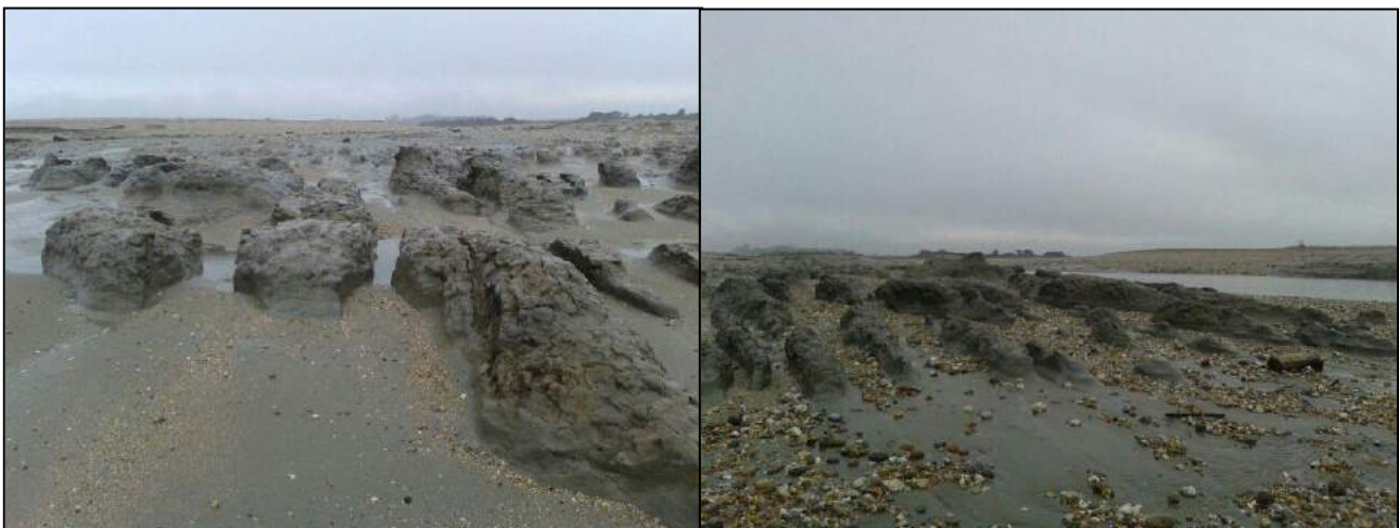
Figure 18: Exposed ‘mudstone’ at Medmerry (CCO, 29/10/2014)
